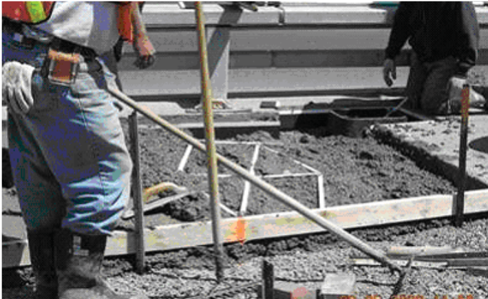
Installation of counter sensors on Alexandra Bridge May 2009
