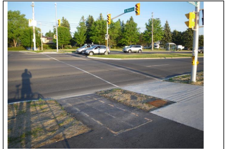
View from Riverside Drive/Mooney's Bay path at the Walkley intersection. Approach to pedestrian crosswalk is concrete; ramp for bikes to cross and ride east on Walkley is asphalt. Markings for the bike sensor loop to activate the signal are visible. Photo: CfSC
