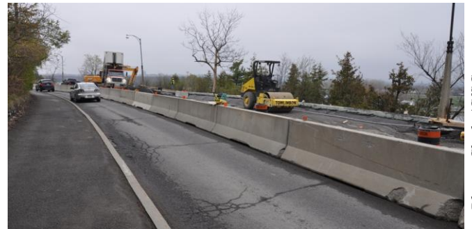
Rockcliffe Parkway under construction. Photo: Clarke/CfSC
