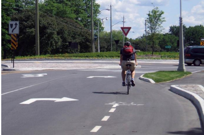
Southbound approach to the Prince of Wales-Experimental Farm roundabout. Photo: Clarke/CfSC
